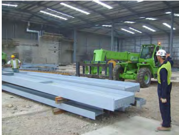
Figure 19 - Use of Wider Fork Carriage
