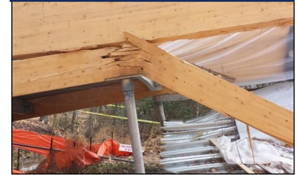
Case Study 9 : WAKE TECH BRIDGE COLLAPSE?
