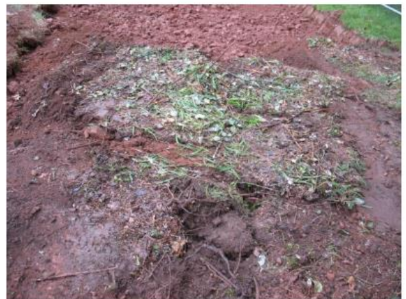
Turf after placing and light consolidation
