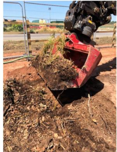
Removal of turf from donor site, containing bracken stems
