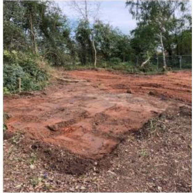
Donor soil in foreground awaiting removal and stripped donor site in background
