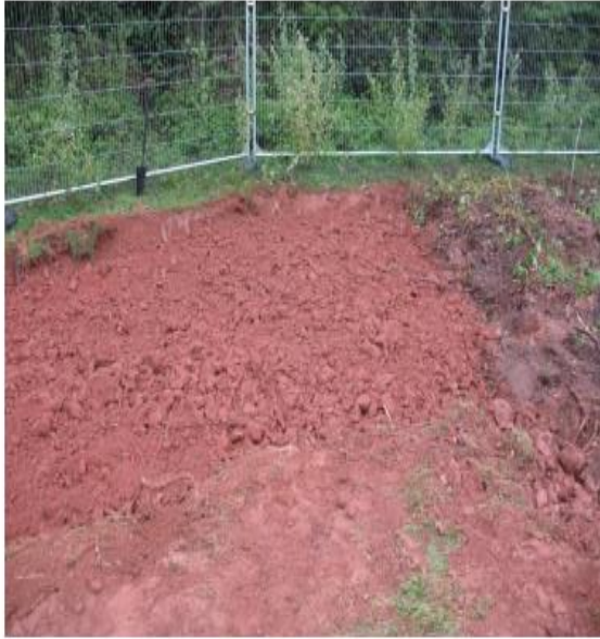
Prepared receptor site following loosening of subsoils with landscape rake
