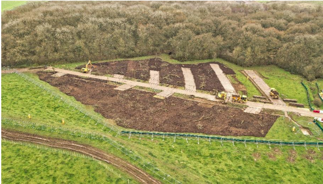
Aerial view of receptor site during works, looking to south, Decoypond wood in background. Track mat system visible in photo, with mats removed as areas completed
