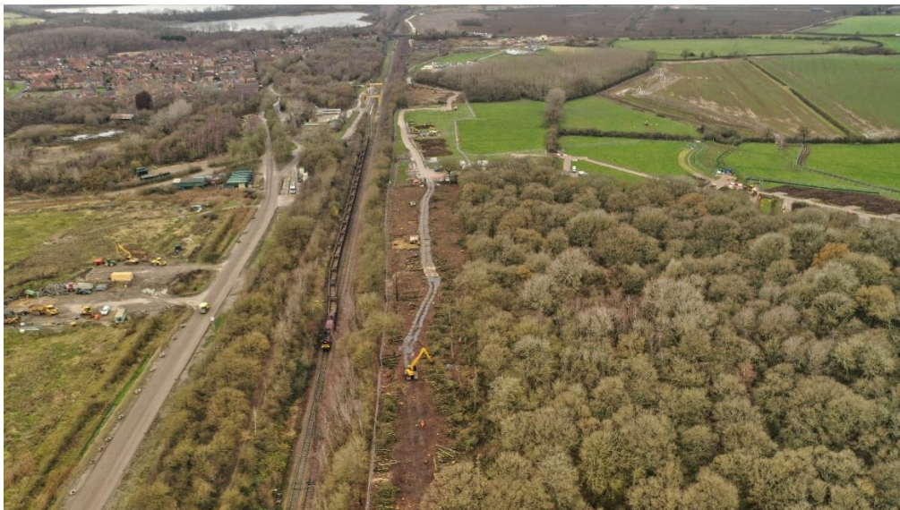
Decoypond Wood donor site (DT06) during felling and translocation works
