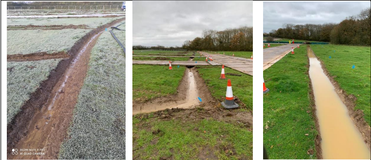
Above: Network of grips at edges of cells connect to central channels positioned left and right of main haulage route
