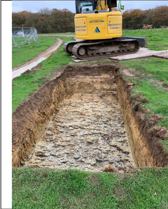
Above: Excavation of area on northern boundary to create drainage sump
