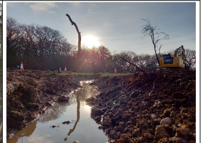
Above: Reprofiled drainage ditch at receptor site – will act as semi-permanent wet feature during heavy rainfall
