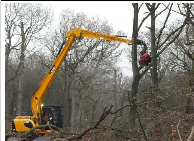
Above: Excavator removing a section of tree with shears
