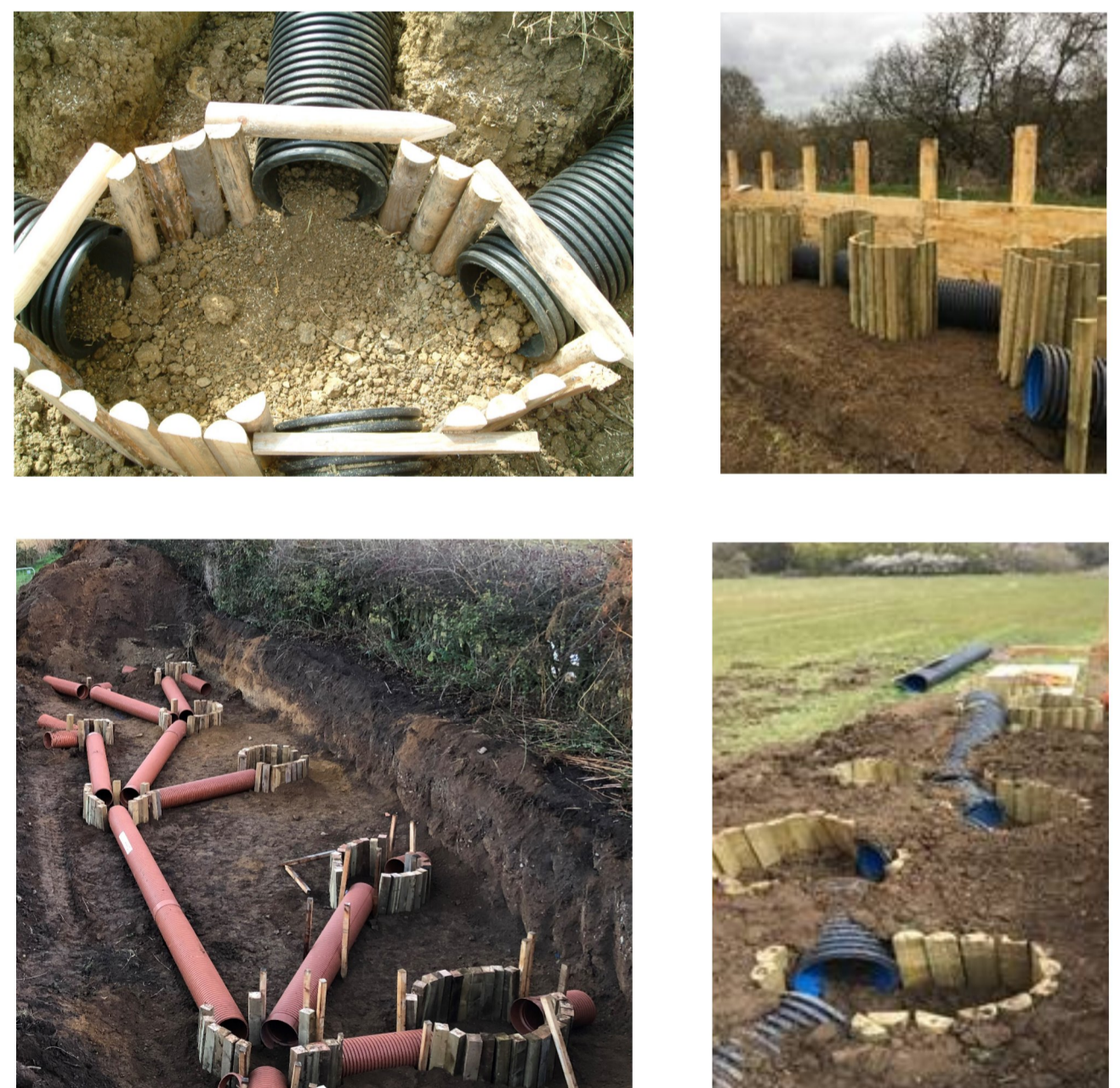
Example badger sett construction images - illustrative only as chamber construction may vary from site to site - see notes.
