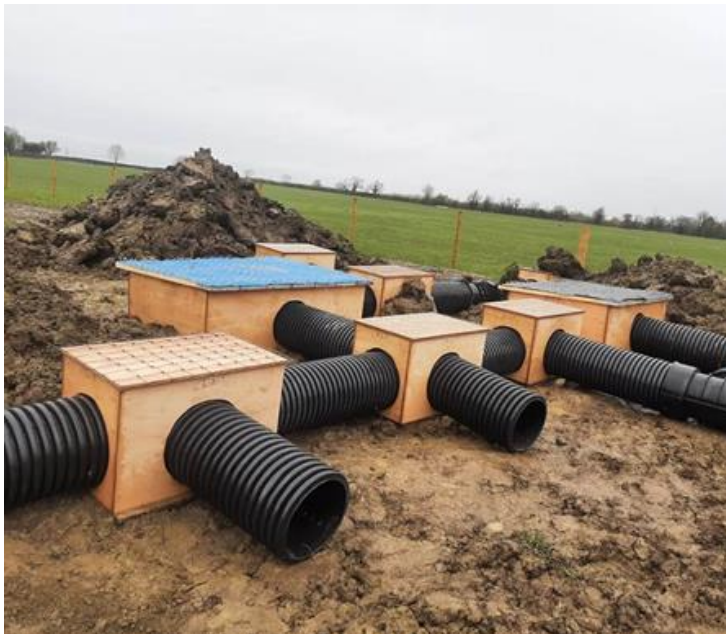
Figure 3: ABS remediation. New sett replacing failed ABS which used plastic pipes but retained use of FSC plyboard for chambers (left). Test design for ABS entrances on non-HS2 sites, as part of the on-going process of improving the sustainability of ABS design (right). Photos courtesy of SES.
