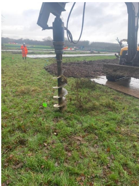
Above left: Auger attached to excavator preparing pit
