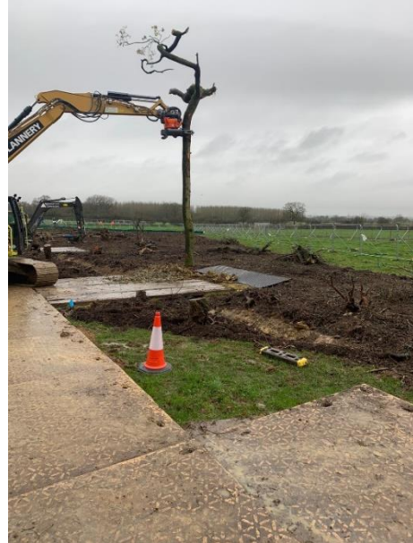
Above right: Monolith being lifted into position
